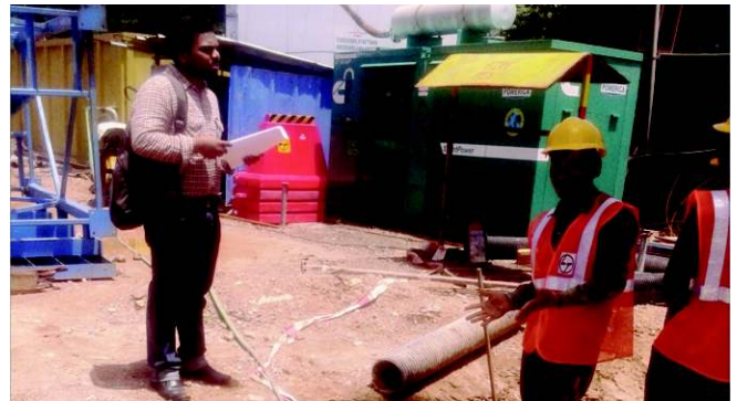
Interaction with migrant labours in a construction site
