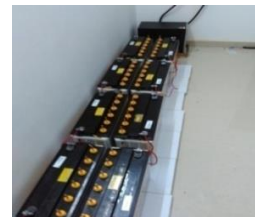
Battery bank for 2kw solar power plant at private Residence at Thakazhi
